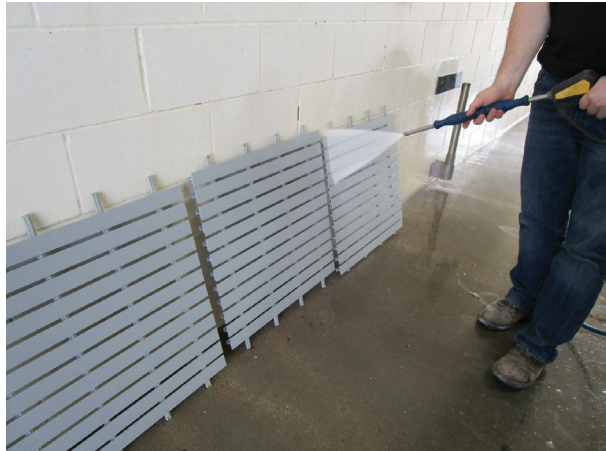
Figure 10 – Pressure washing grating panels.
