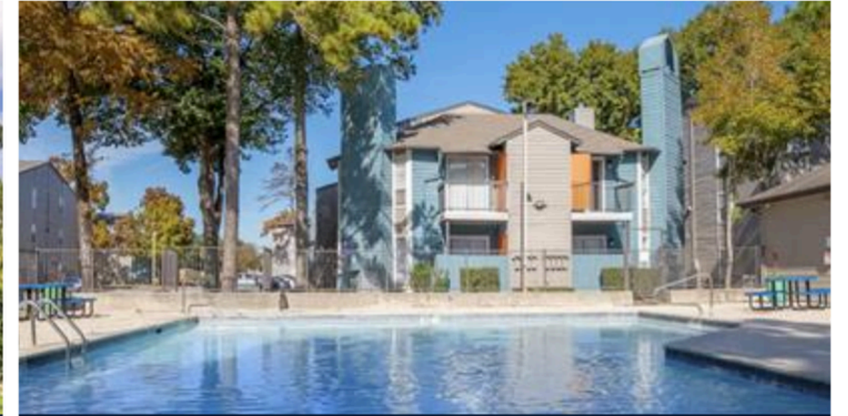
Cranbrook Forest 261 Units – Houston, TX
