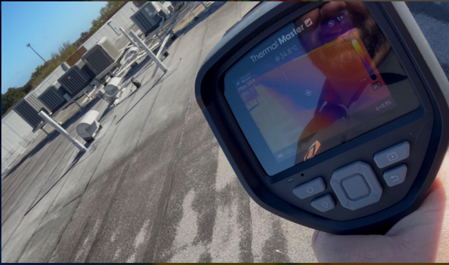
Infrared cameras detect heat differences that often signal moisture trapped within insulation layers.
