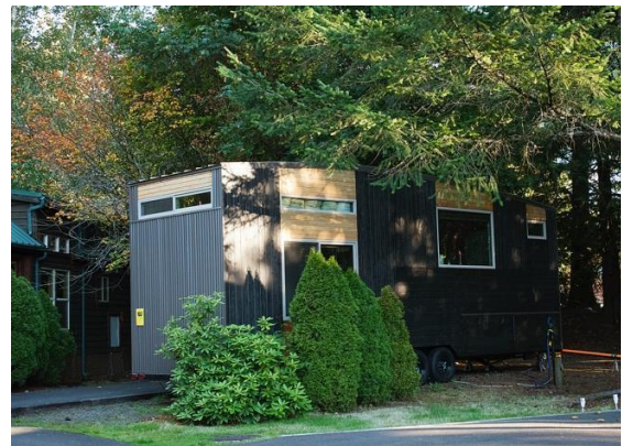
Fig 4. Tiny house connected to utilities with vegetative screening
