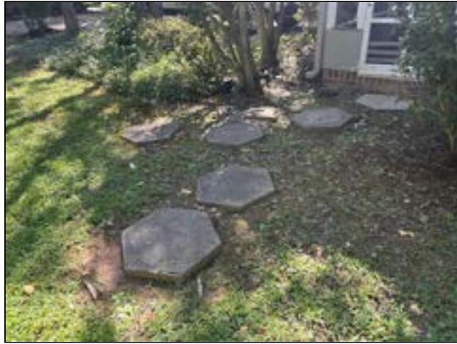
2.4 Item 6 (Picture) Be aware of potential trip hazards at the walkway(s). Correction is recommended for safety
