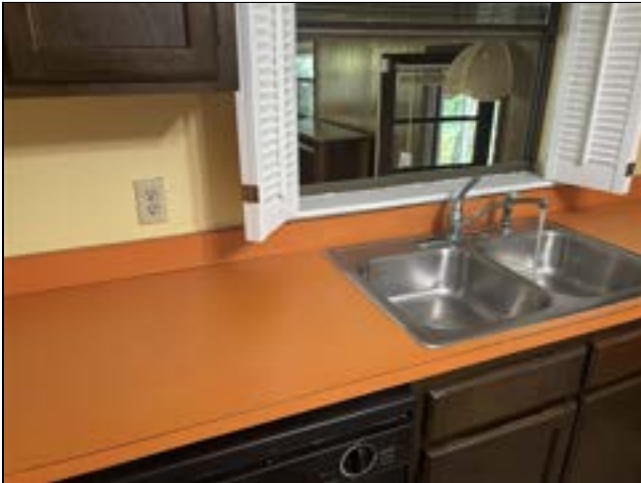
7.4 Item 1 (Picture) All kitchen receptacles serving countertops should be GFCI protected and are not (regardless of proximity to sink). While this was not required when the house was built, it is a potential safety hazard. I recommend having a qualified electrician correct as a safety upgrade.
