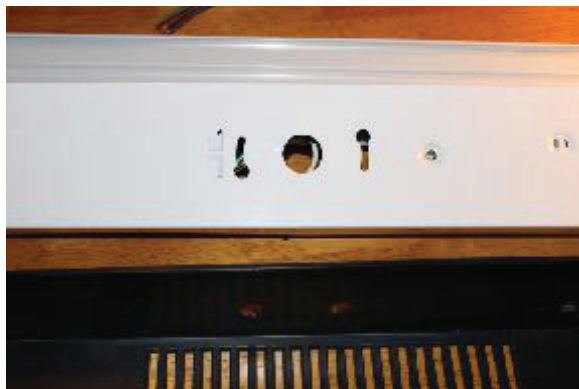
Knock out port in new unit to accept the power cable.
