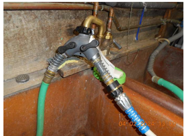
Y faucet adapter. Tub hose on left, aquarium hose on right
