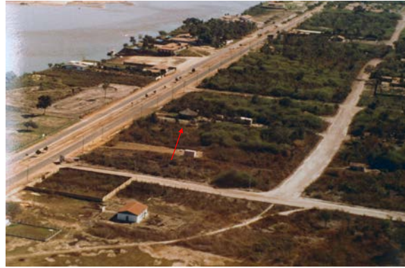
Aerial view of Luis' home, with Rio Vermelho across the street.
