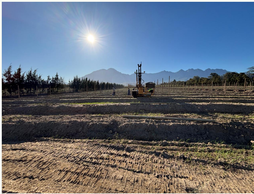
FIELD APPLICATION / VINEYARD POST INSTALLATION
