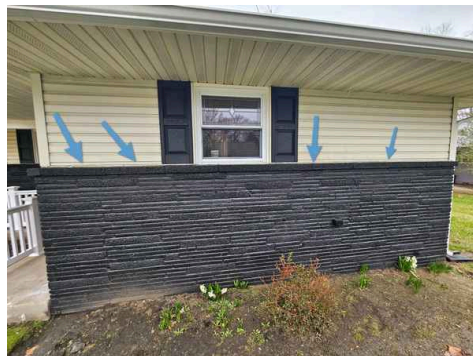
Front - Along the front edge where the vinyl siding meets the stone veneer.
