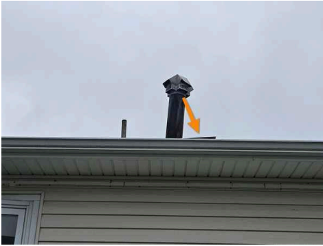
Pushing the shingles up preventing water from discharging off the roof.
