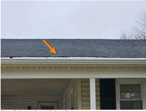
Pushing the shingles up preventing water from discharging off the roof.
