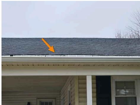
Pushing the shingles up preventing water from discharging off the roof.
