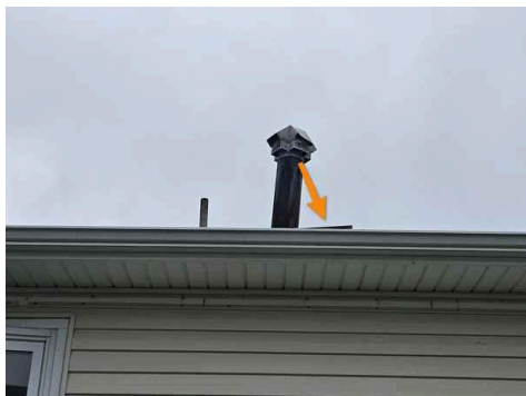
Pushing the shingles up preventing water from discharging off the roof.
