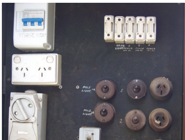
Zelemite backing board to an external switchboard
