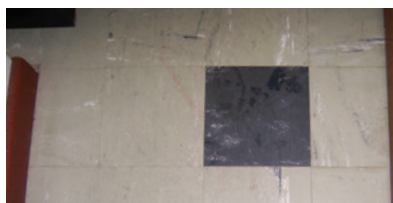
Vinyl floor tiles
