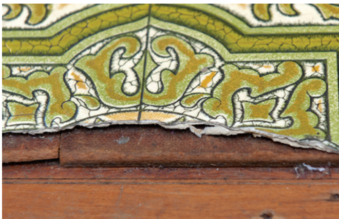
Asbestos backed vinyl sheet flooring
