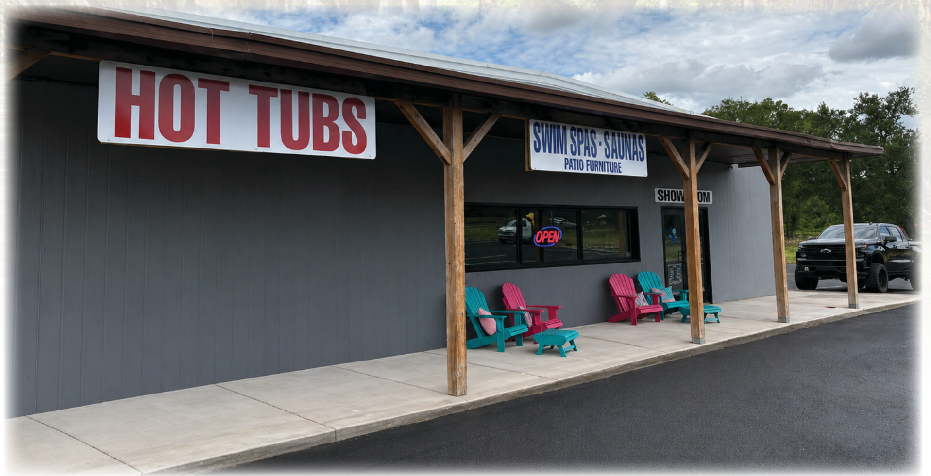
The entrance to Paradise Patio Solutions in Bushnell. They specialize in helping homeowners create the perfect backyard retreat with high-quality spas, saunas and even patio furniture.
