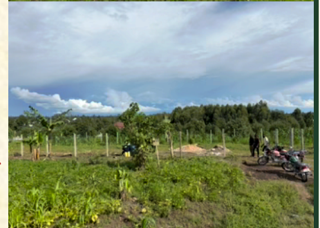
Putting up the poles in Bwera
