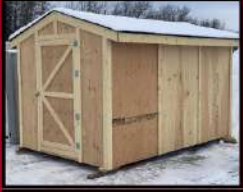
UNUSED 8 FT X 12 FT SHED
