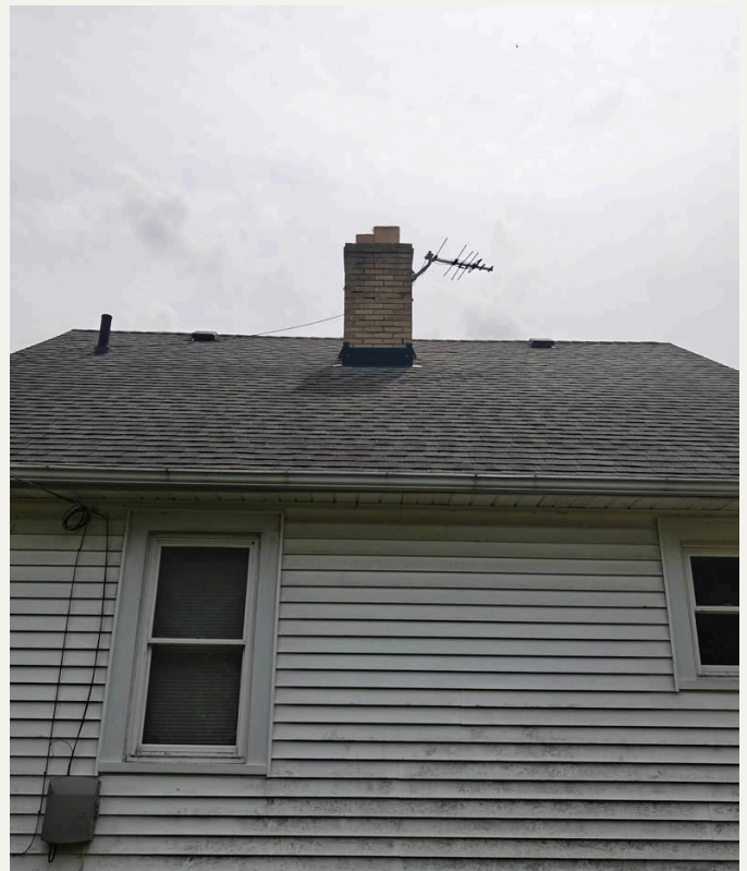
Asphalt shingle roof and chimney
