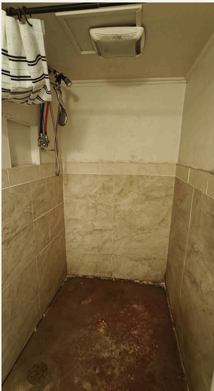
Basement tiled shower stall, second full bath
