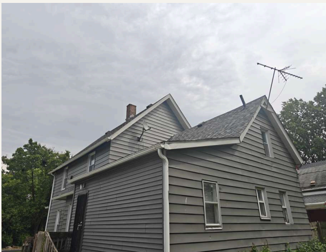
Side and rear elevation, brick chimney
