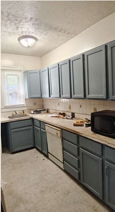
Lower unit kitchen, sink wall
