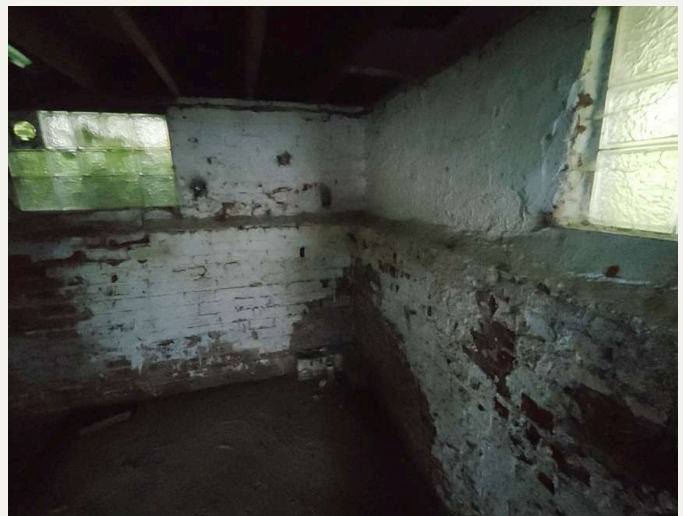
Basement wall, brick foundation
