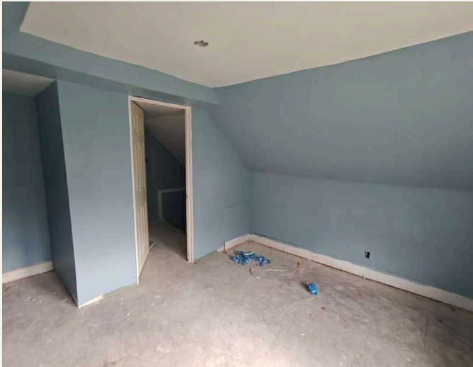
Third floor room under the roof
