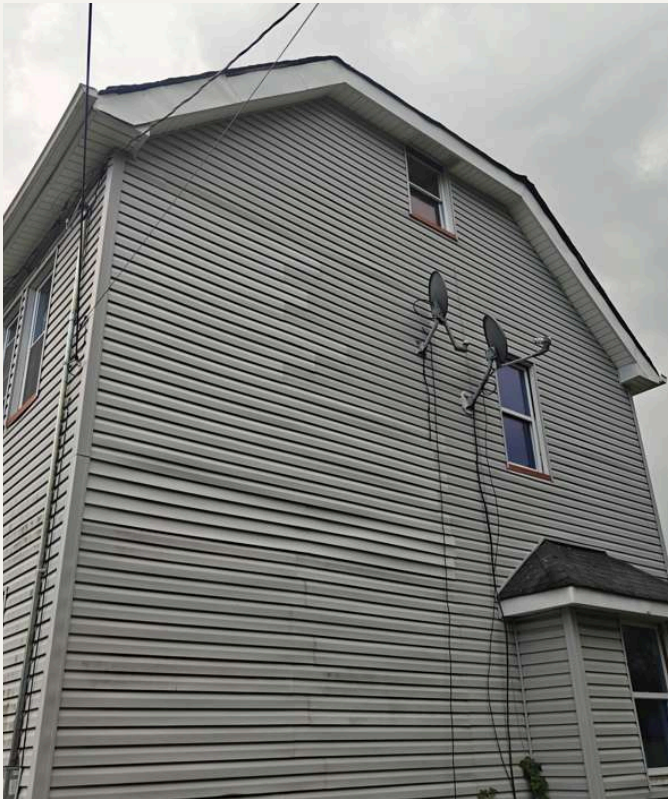
Side and rear elevation, roof over the rear entry
