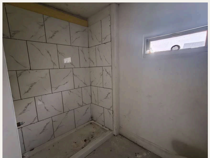
Bath, shower base and partial tile surround
