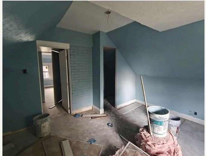
Third floor, painted brick chimney and closet
