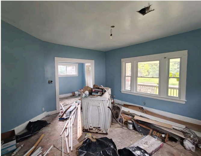
Living room, windows to the front porch
