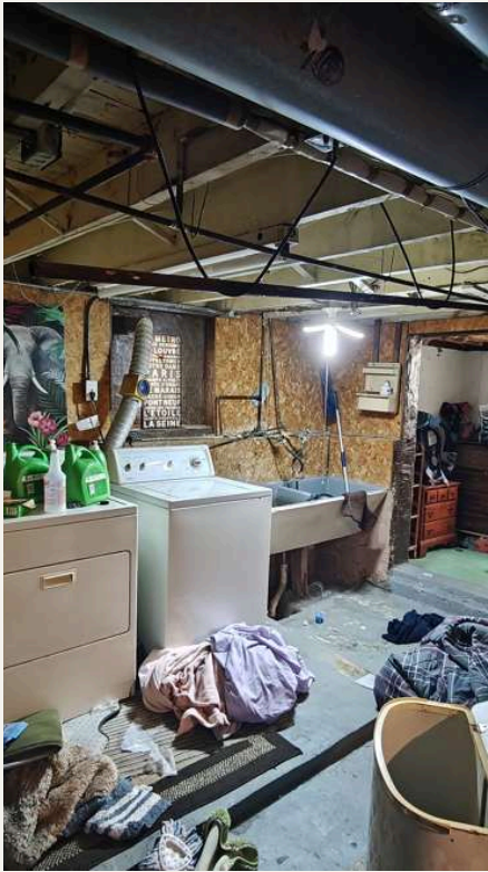
Basement, laundry tub and washer and dryer hookups
