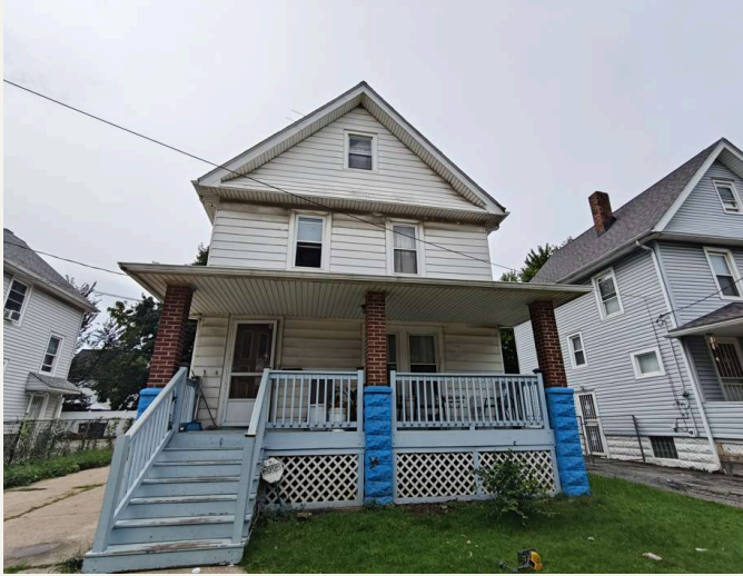
Front elevation from Stevenson Rd
