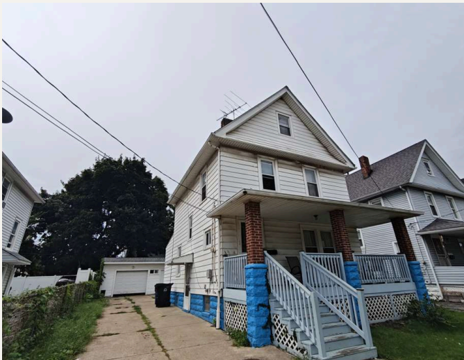
Side elevation, driveway, and garage at the rear
