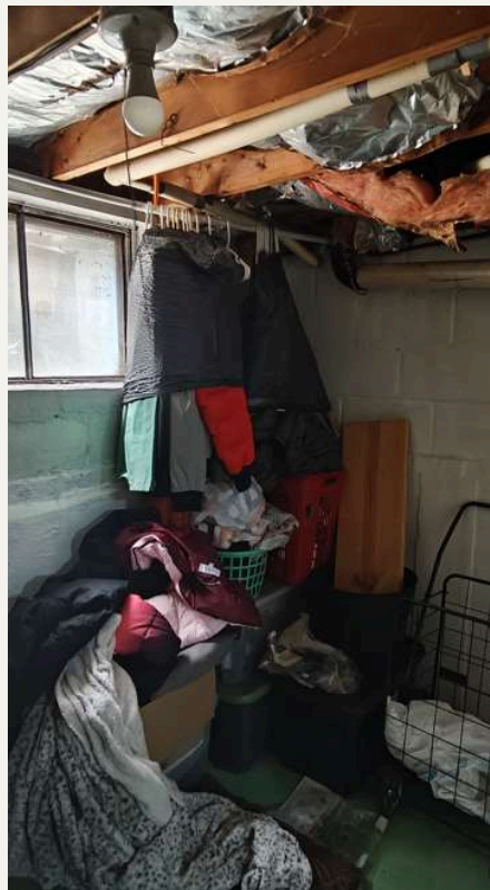
Basement, block foundation walls
