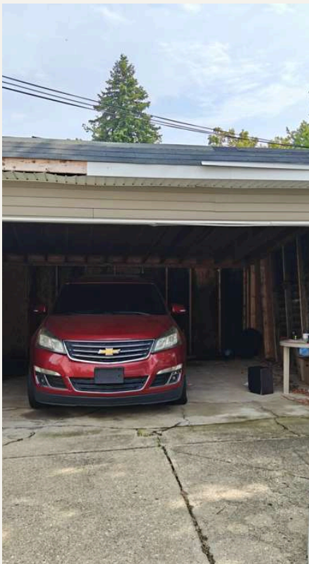
Detached two-car garage at the rear of the drive
