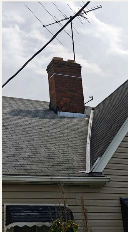
Roof, chimney, and front awnings
