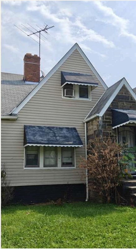
Front elevation from E 149th St
