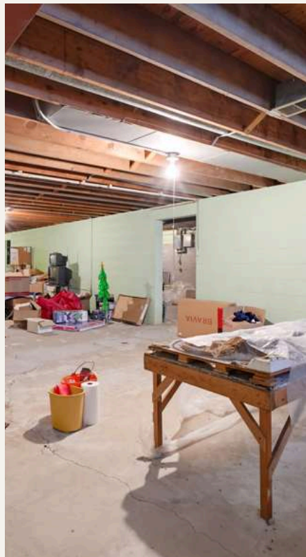
Basement main area
