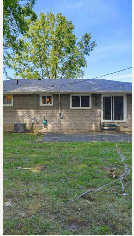
Rear elevation and patio
