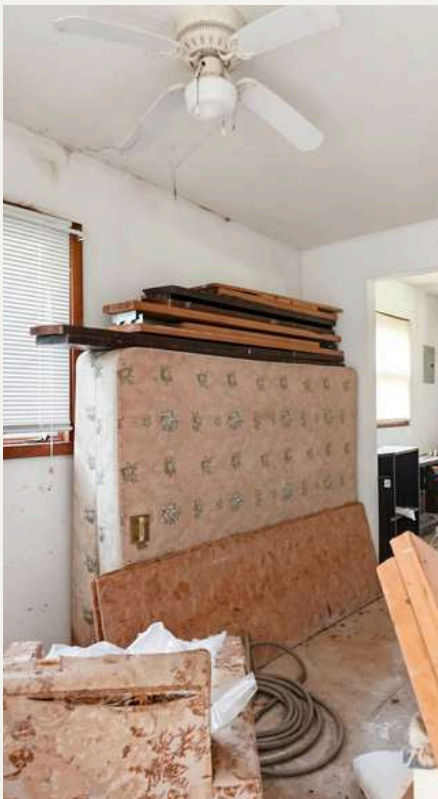
Additional structure, interior.
