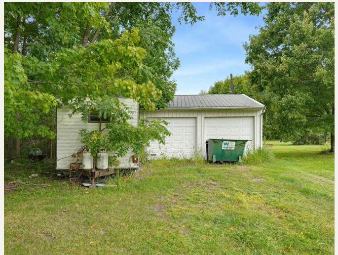
Garage and shop.
