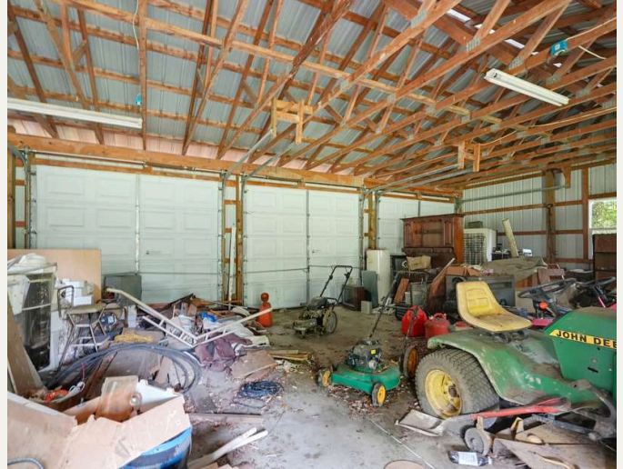
Pole building interior.
