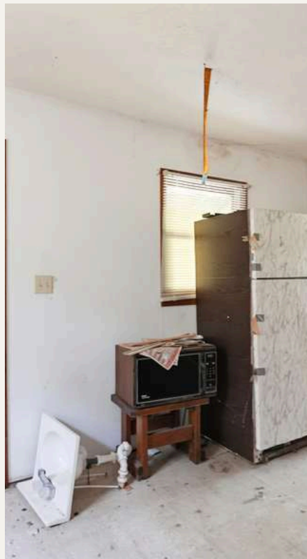
Additional structure, interior.
