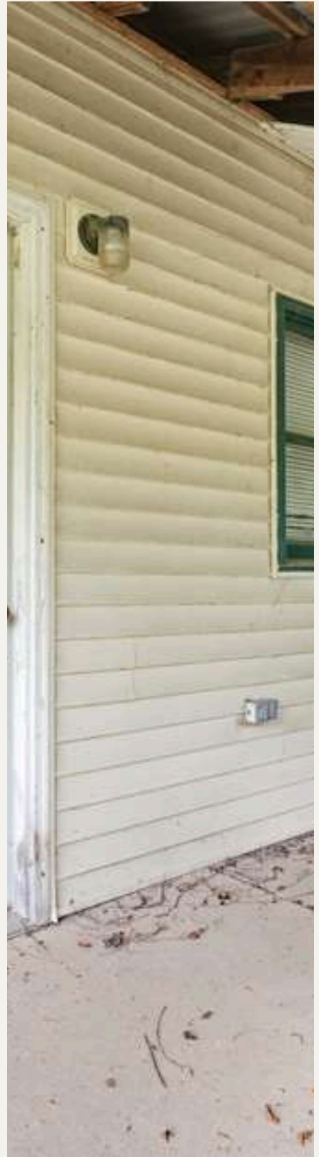
Additional structure, porch.
