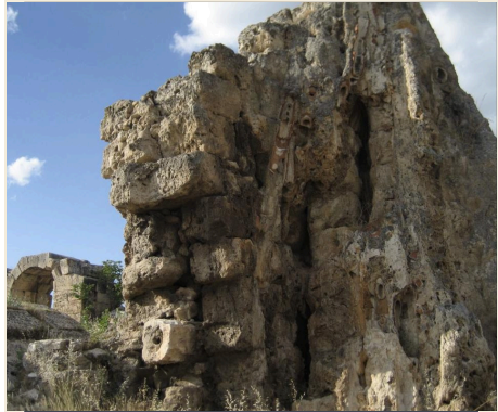
A water tower at Laodicea. The round holes are the ends of stone water pipes, and the white crust is minerals left by the water. Photo Rjdeadly, CC BY SA 4.0.
