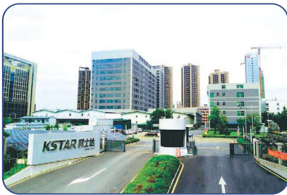
Kstar Industrial Park, Zhongkai High-tech Zone, Huizhou City, Guangdong
