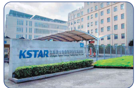
Jiangsu Kstar New Energy Technology Co., Ltd.
