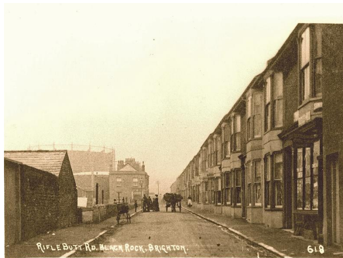
A view of Rifle Butt Road looking north, with the bakery in the middle distance and, to its left, the gasometer.
