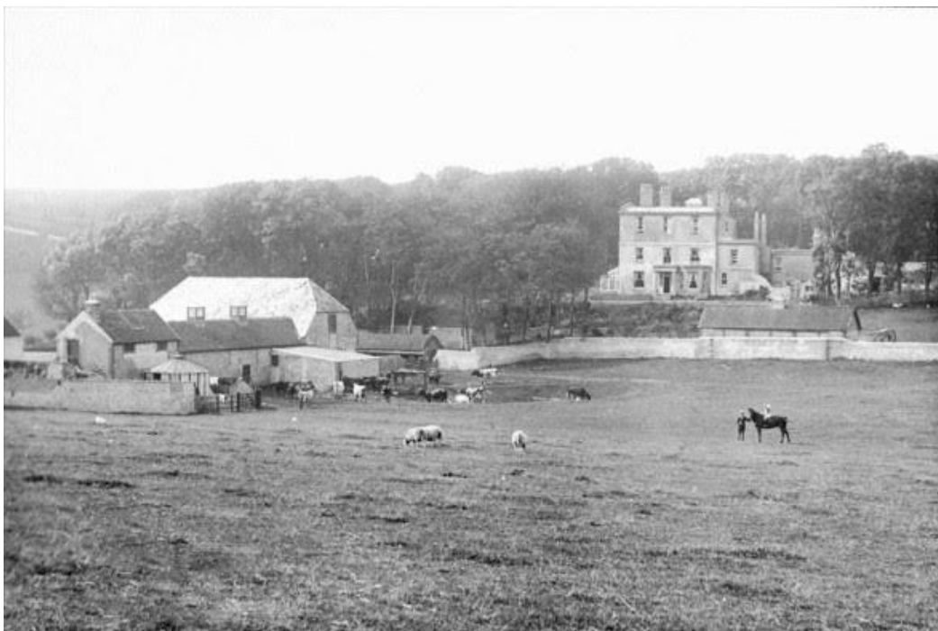
Woodingdean House & Woodingdean Farm, Ovingdean Road, Woodingdean
