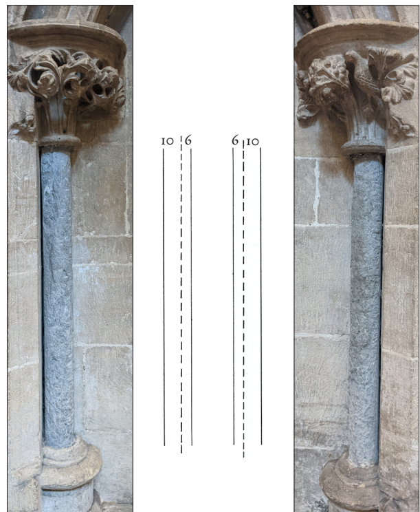
The six foot range stretches between the 8/5 divisions of the pillar's widths
