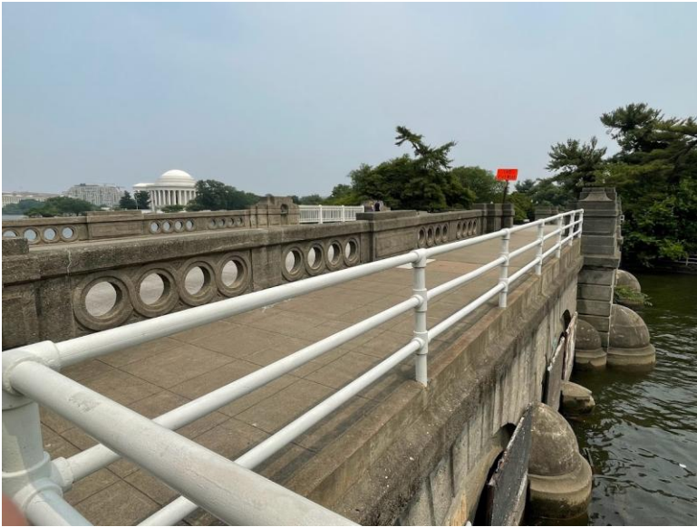
The Inlet Bridge
