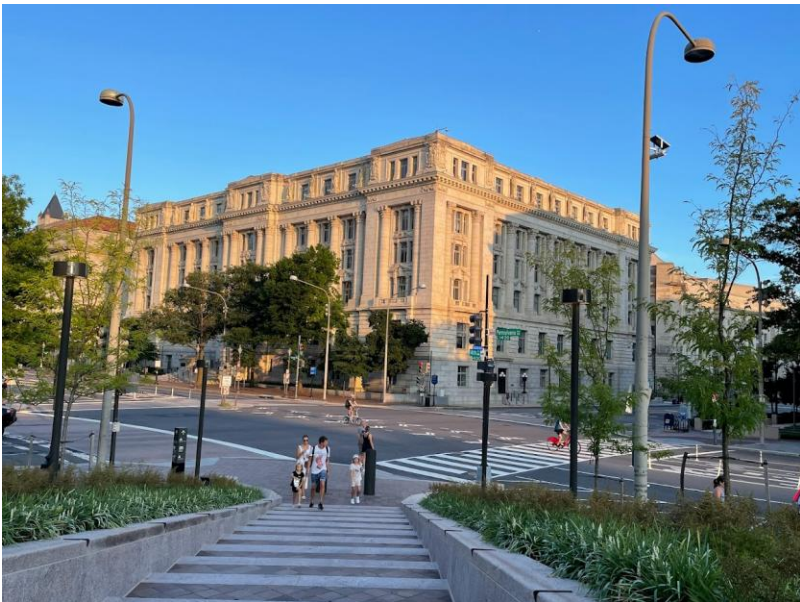
John A. Wilson Office Building
