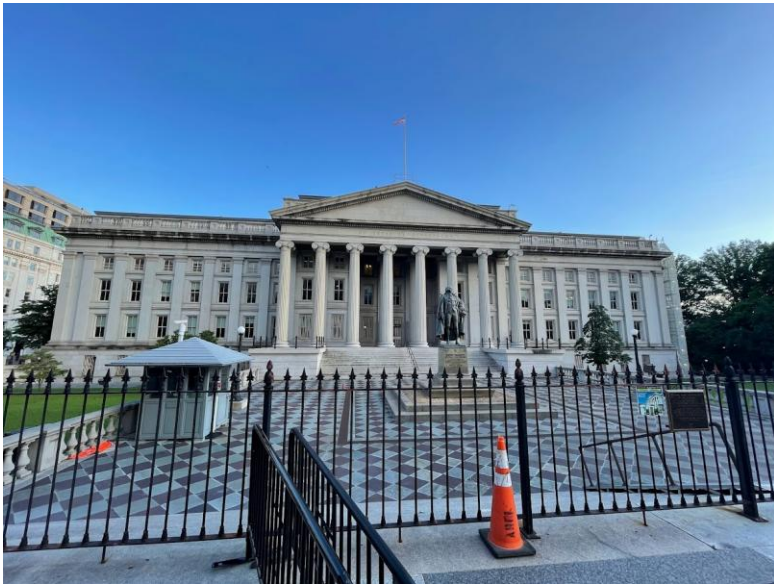
Department of Treasury Building
