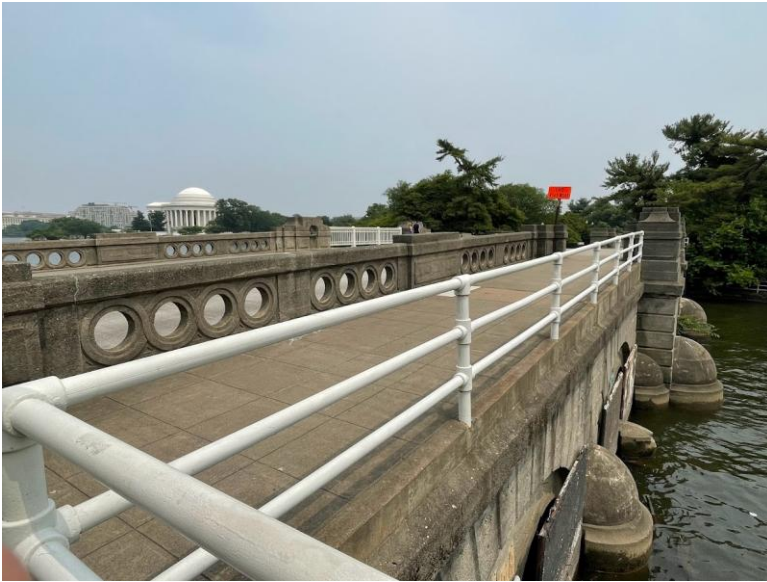
The Inlet Bridge
