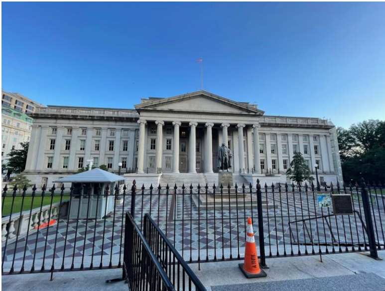
Department of Treasury Building
