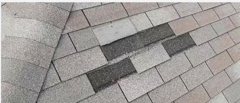
MISSING SHINGLES
