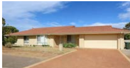
14/179 Canning Highway, South Perth Source: RP Data
