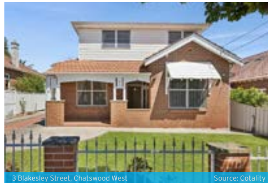
3 Blakesley Street, Chatswood West
