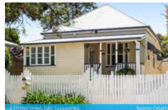
2 Shipley Street, East Toowoomba Source: Cotality
