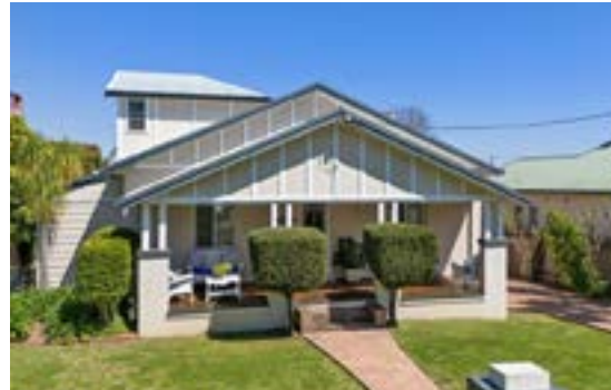
77 Upper Street, East Tamworth
