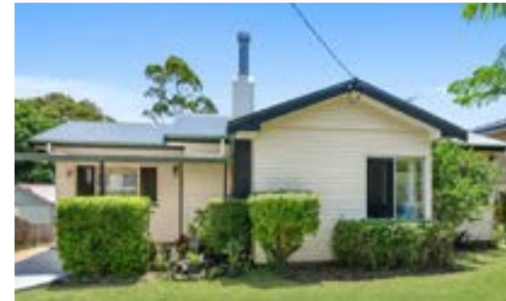
5 Wyndham Street, North Toowoomba
