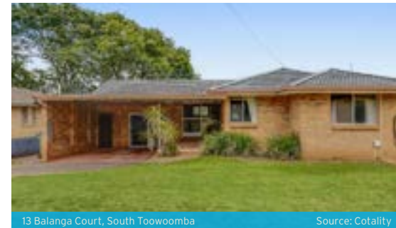
13 Balanga Court, South Toowoomba
