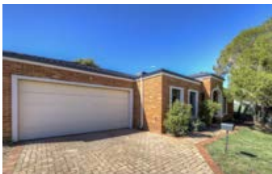
42 Essex Street, Bayswater
