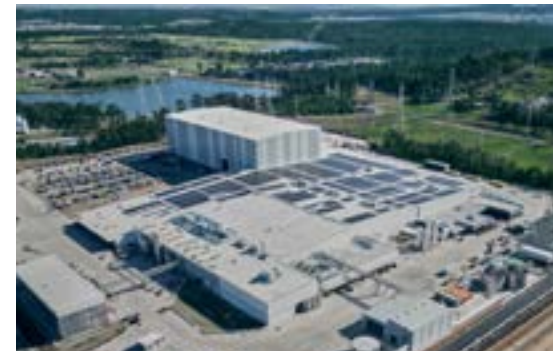
Suntory Oceania's new Ipswich factory
