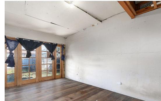
87 Weller Street, Geelong West - before
