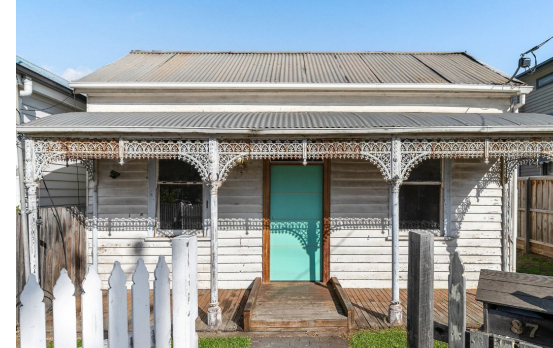
87 Weller Street, Geelong West - before
