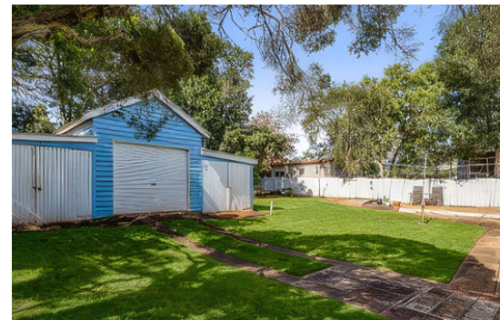
2 Joffre Street, East Toowoomba unrenovated in May 2021
