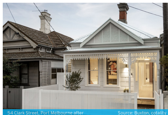
54 Clark Street, Port Melbourne after
