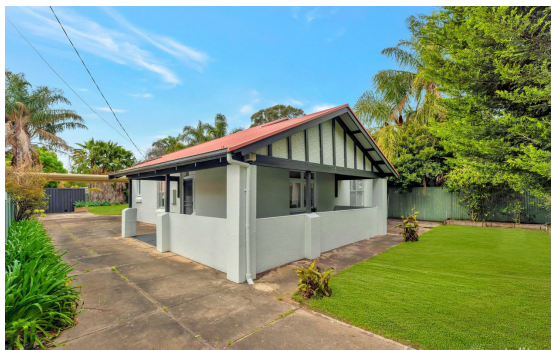
1 Springbank Road - Pre-Renovation Source: realestate.com.au
