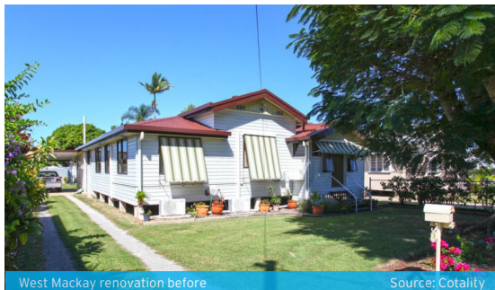
West Mackay renovation before
