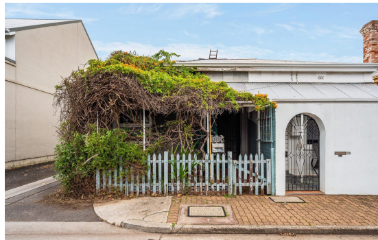
24 Marion Street - Frontage Source: realestate.com.au
