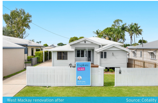
West Mackay renovation after
