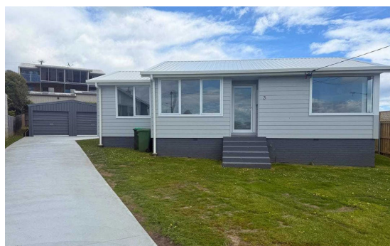
3 Soutar Street, Devonport - after
