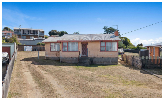
3 Soutar Street, Devonport - before
