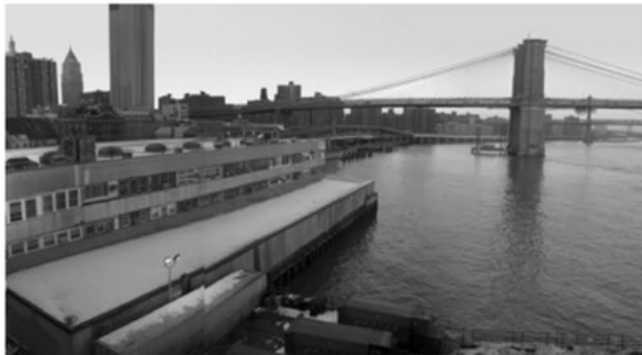
NEW MARKET BUILDING - EXISTING CONDITION
