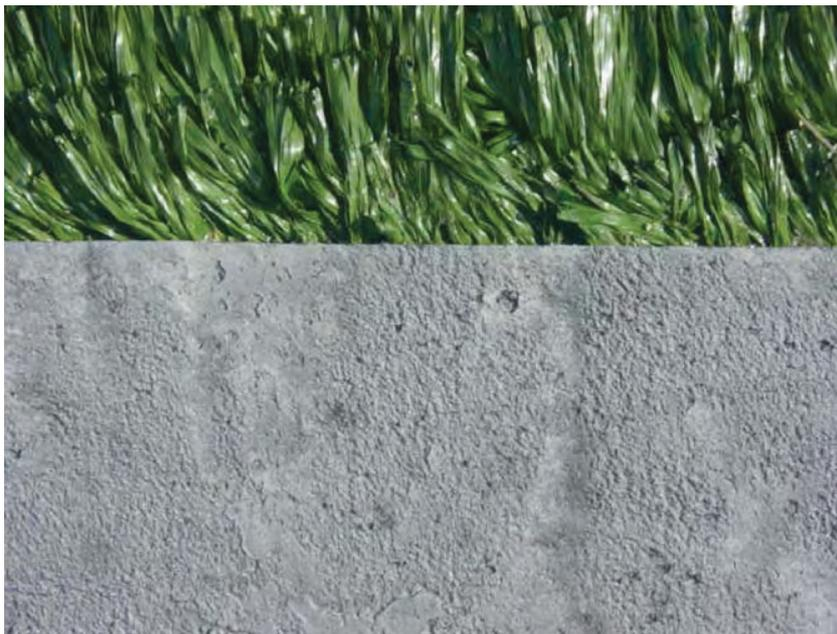
FIGURE C-40. THE 2.0-INCH FIBER WITH QUICK-DRYING CONCRETE HEADER
