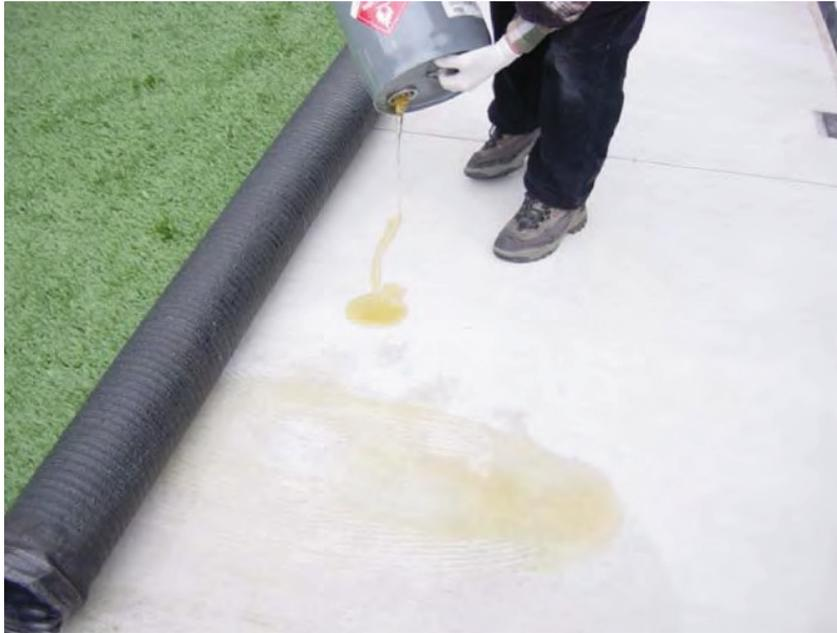
FIGURE C-39. APPLICATION OF ARTIFICIAL TURF TO CONCRETE
