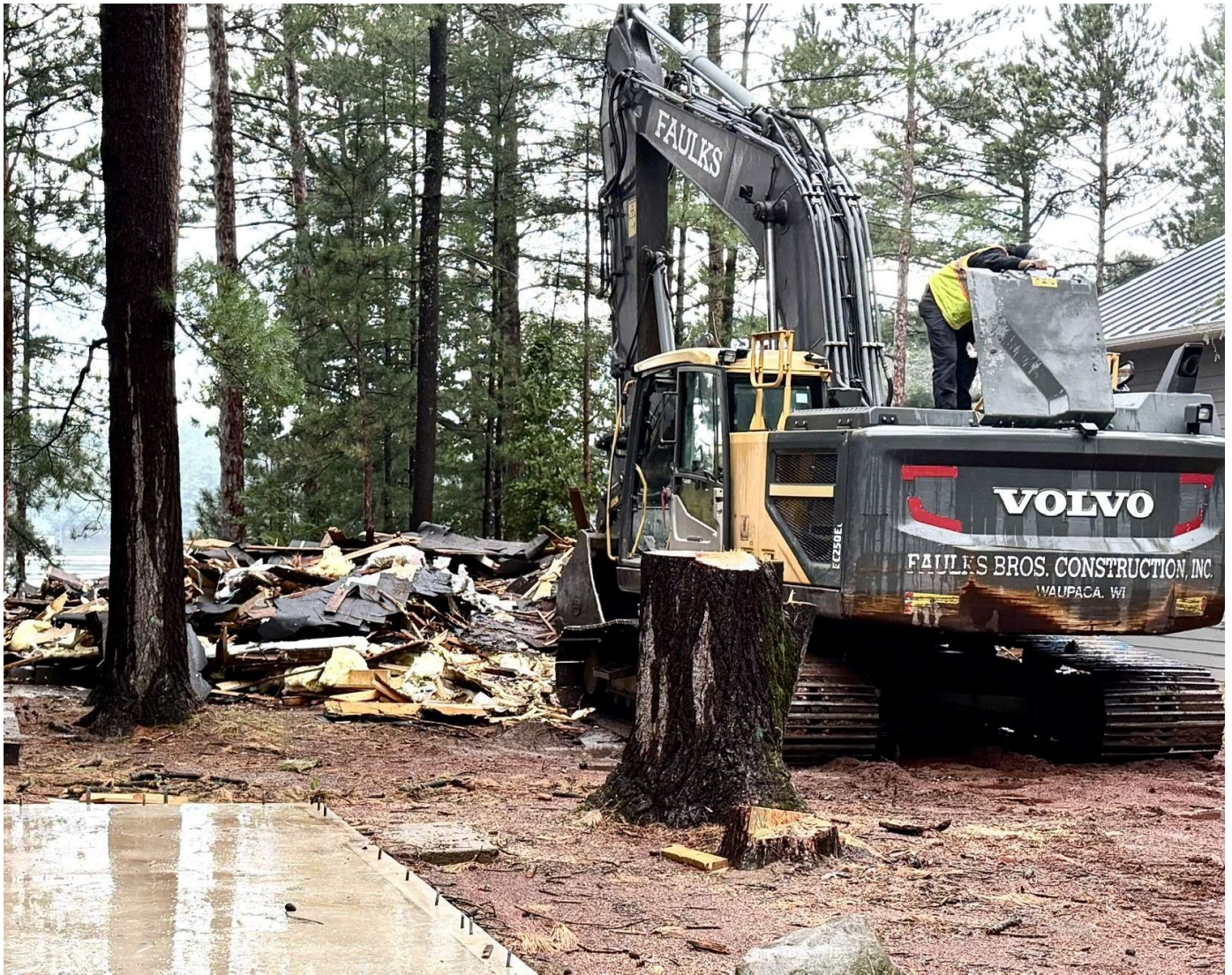
Site preparation and demolition underway for a new Waupaca Chain home.
