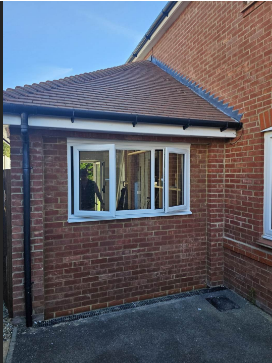
Completed external frontage with new window, matched brickwork and drainage channel.
