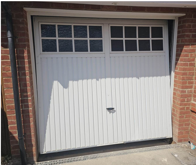
The original up-and-over garage door before the front elevation was rebuilt.
