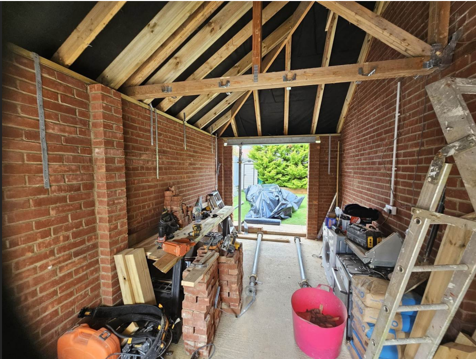
The stripped garage shell exposed the existing roof, masonry and load paths for review.
