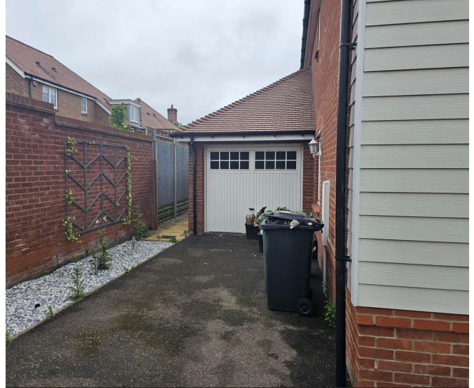
The existing single garage viewed from the driveway before conversion.
