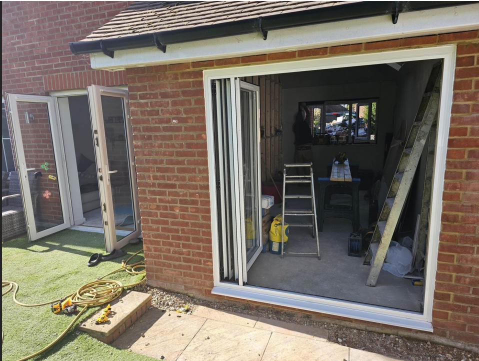
JB Building Projects supplied and fitted the bifolding doors to the new garden opening.
