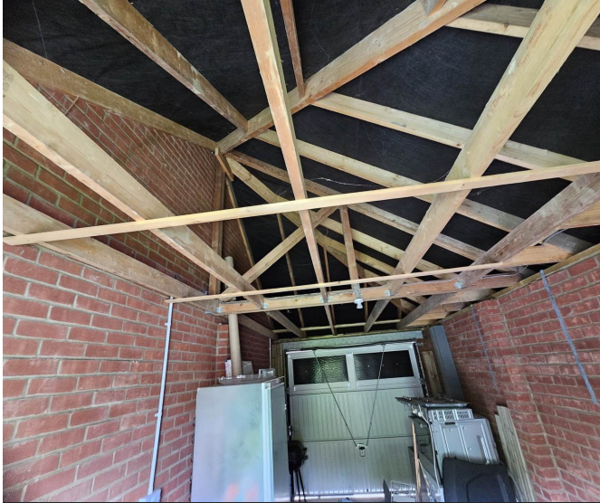
The original unlined shell, exposed roof structure and garage-use finishes.
