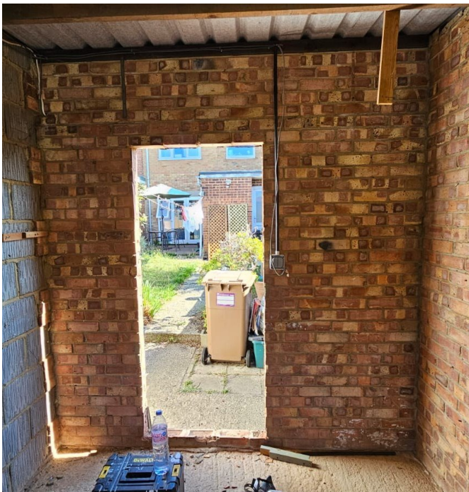
The original rear doorway before the new combined door-and-window opening was formed.
