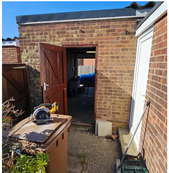
The original external timber door and rear elevation before structural alteration.
