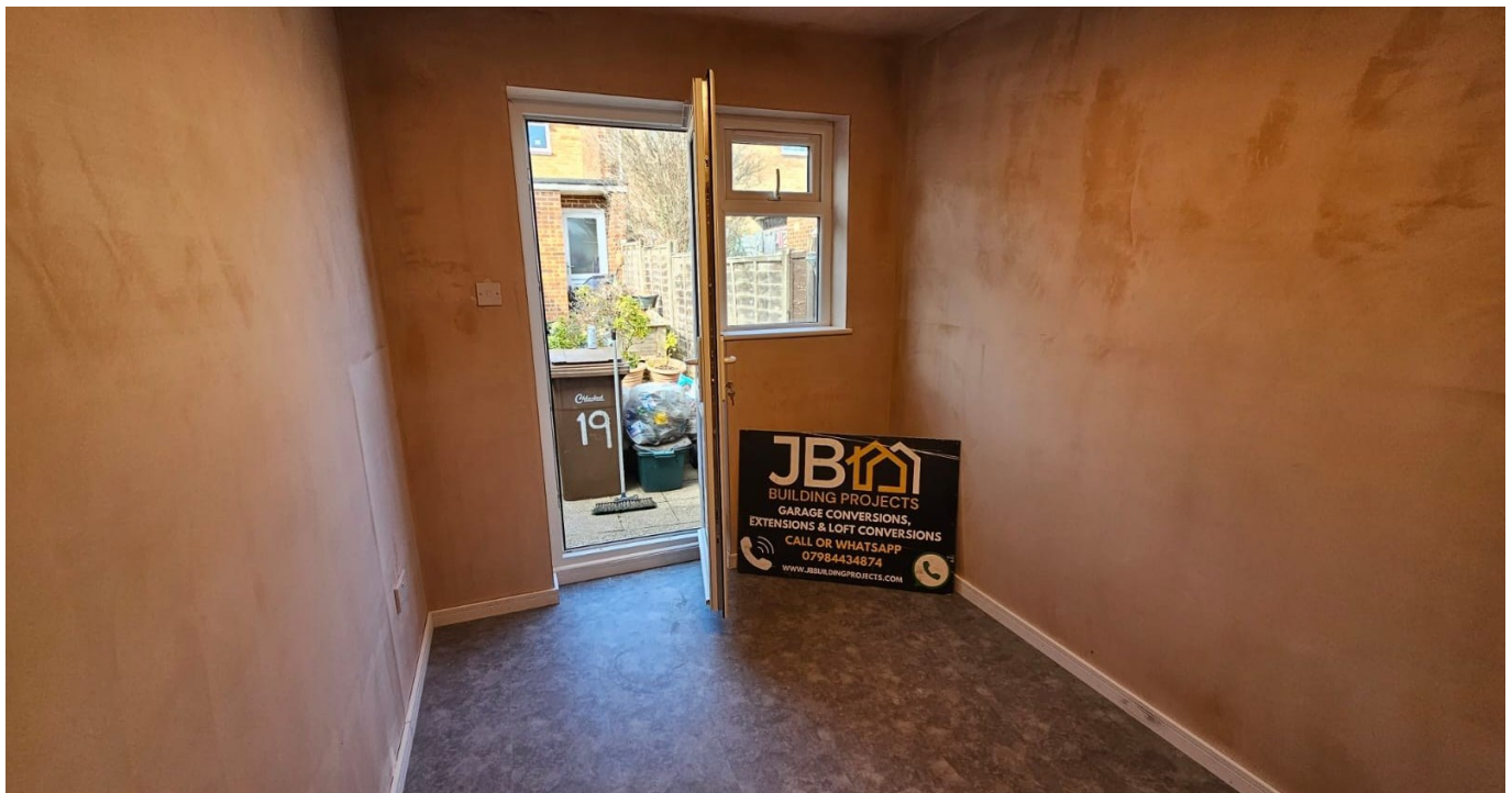
The finished internal room: plastered surfaces, completed joinery, floor finish, lighting and the new garden opening.
