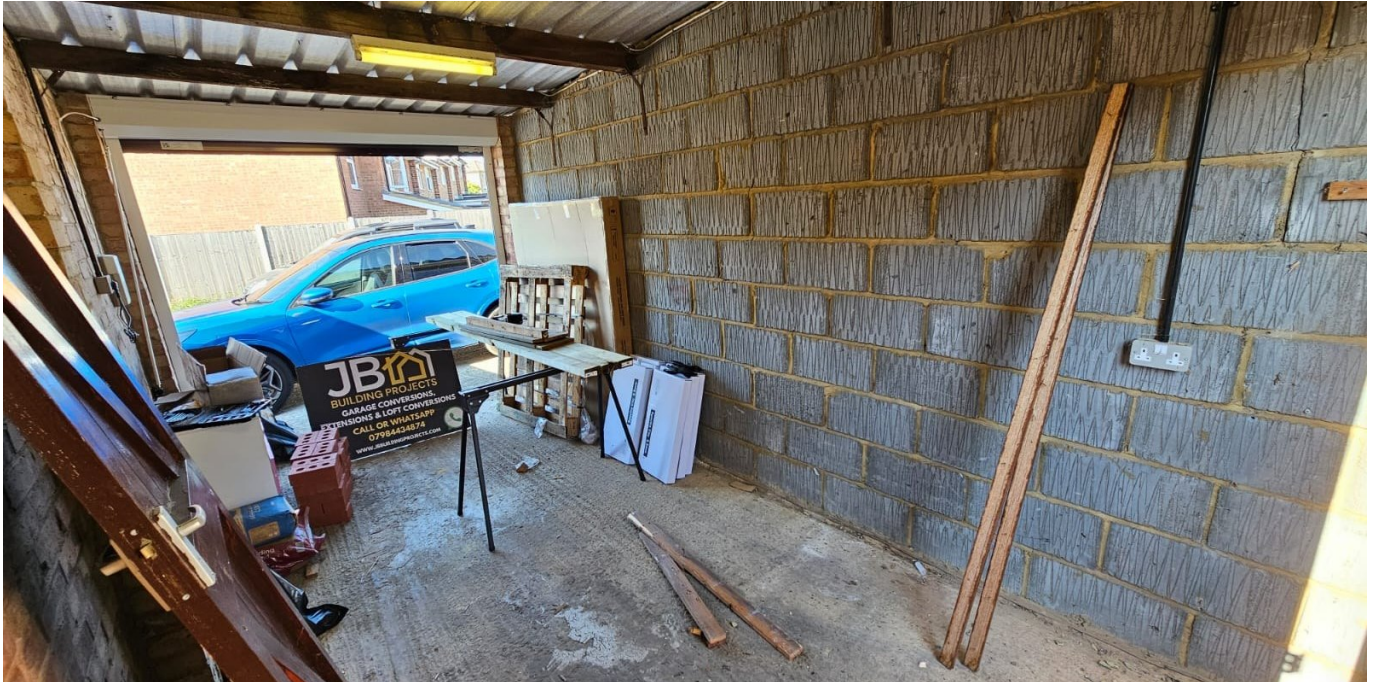
The full garage before zoning: hard floor, exposed blockwork and a roof designed for storage rather than living use.
