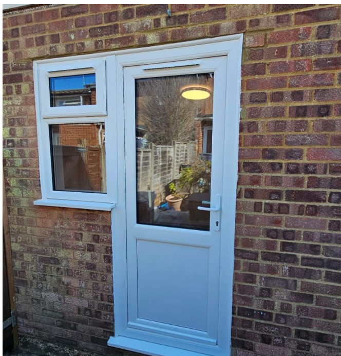
The former timber doorway became a coordinated PVC door and opening window.
