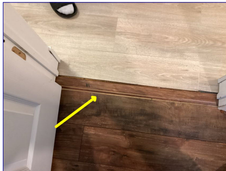
FLOOR FALLING SHORT OF SADDLE
