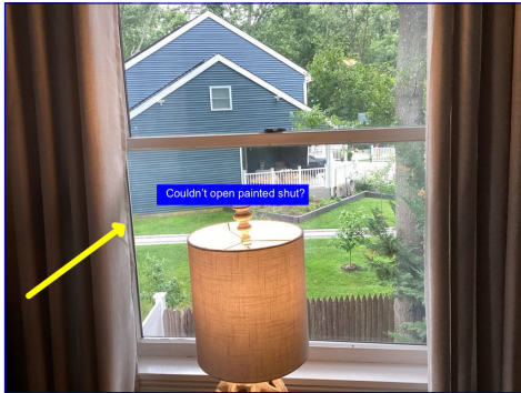
COULDN'T INSPECT PAINTED CLOSED
