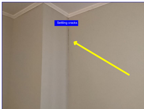
SETTLEMENT CRACKS
