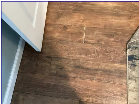
LAMIANTE FLOOR SEPERATING
