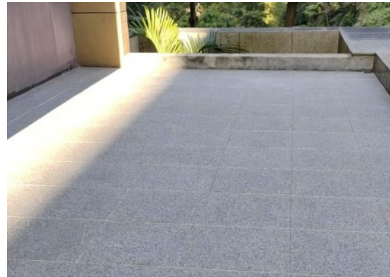
FLAT ROOF - AFTER CLICKTILE INSTALLATION
