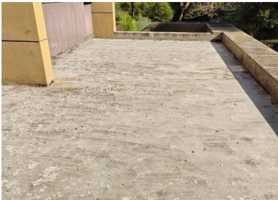
FLAT ROOF - BEFORE CLICKTILE INSTALLATION
